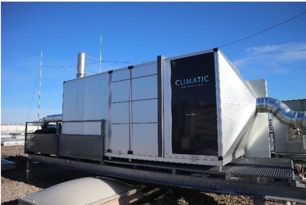
Figure 3: CLIMATIC installation for max. 25,000 m<sup>3</sup>/h (2017).
