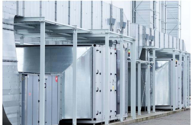
Figure 4: Two UVR-WAC installations for a combined flow of 85,000 m<sup>3</sup>/h (2017).
